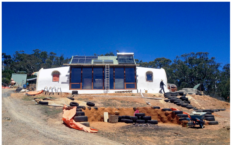
↑ Martin's almost-completed earthship in Ironbank, in the Adelaide Hills, South Australia. The design is based on the Simple Survival Model, adapted for use in Adelaide's warmer climate. The north-facing greenhouse sits in front of the main room which serves as bedroom, living area and kitchenette. An airlock entry room is at the east end of the greenhouse, and a bathroom at the west.
