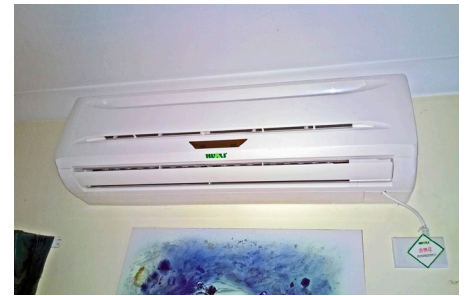
↑ The indoor fan coil unit looks a lot like a reverse-cycle air conditioner.
