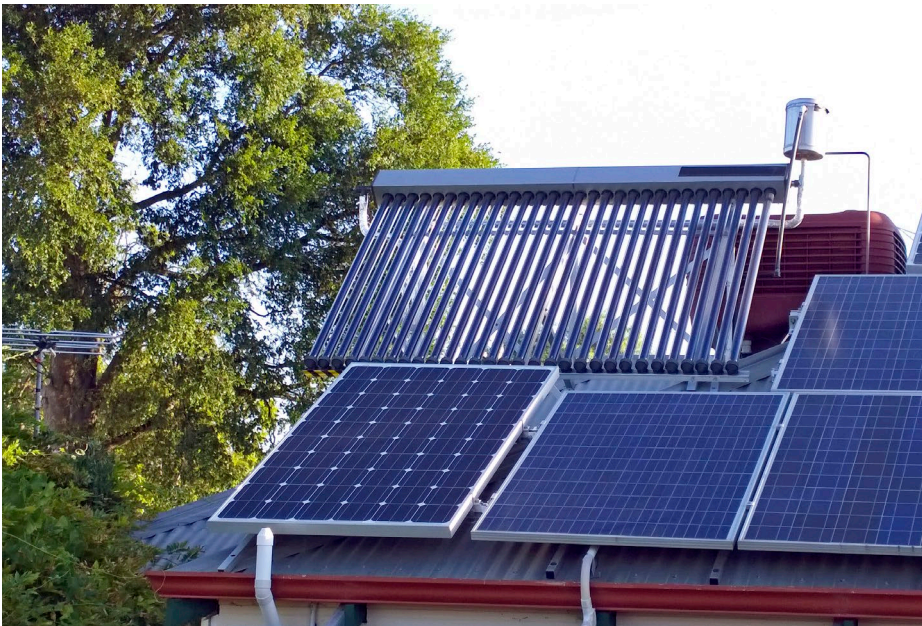
↑ The solar thermal collector (at rear) that provides the heat for the mini hydronic system.
