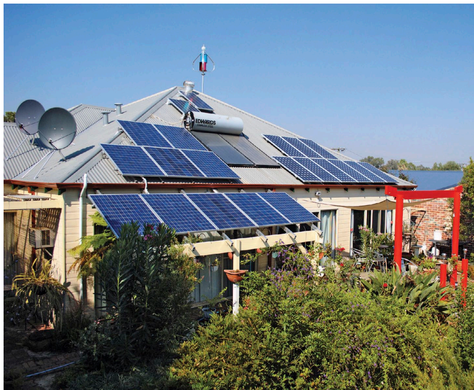
↑ Running out of roof space! Martin has both 12 and 24 volt power systems, solar hot water and a wind turbine.
