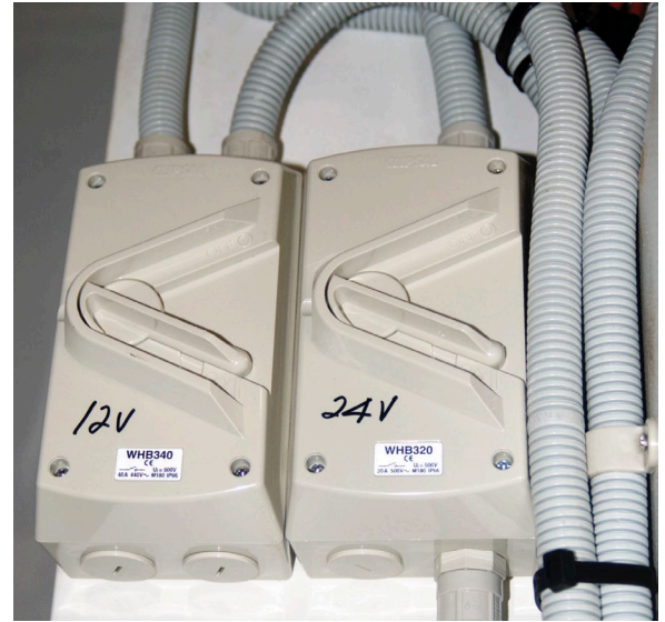
↑ Isolation switches on the solar panels are important safety devices.
