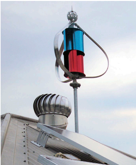
↑ The vertical axis wind turbine. They are much quieter than most horizontal axis machines.
