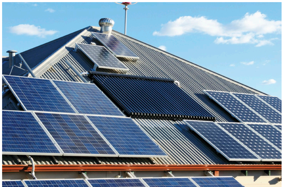
↑ The new evacuated tube panel sits neatly between the (many!) PV arrays.
