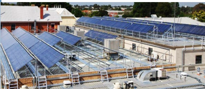
↑ EchUCA Hospital's solar cooling system uses 400m 2 of evacuated tube collectors to heat water for the absorption chiller to generate cooling.
