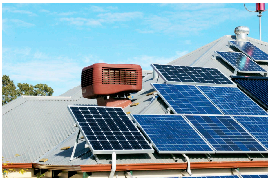
↑ The converted evaporative cooler is powered by two of the solar panels.
