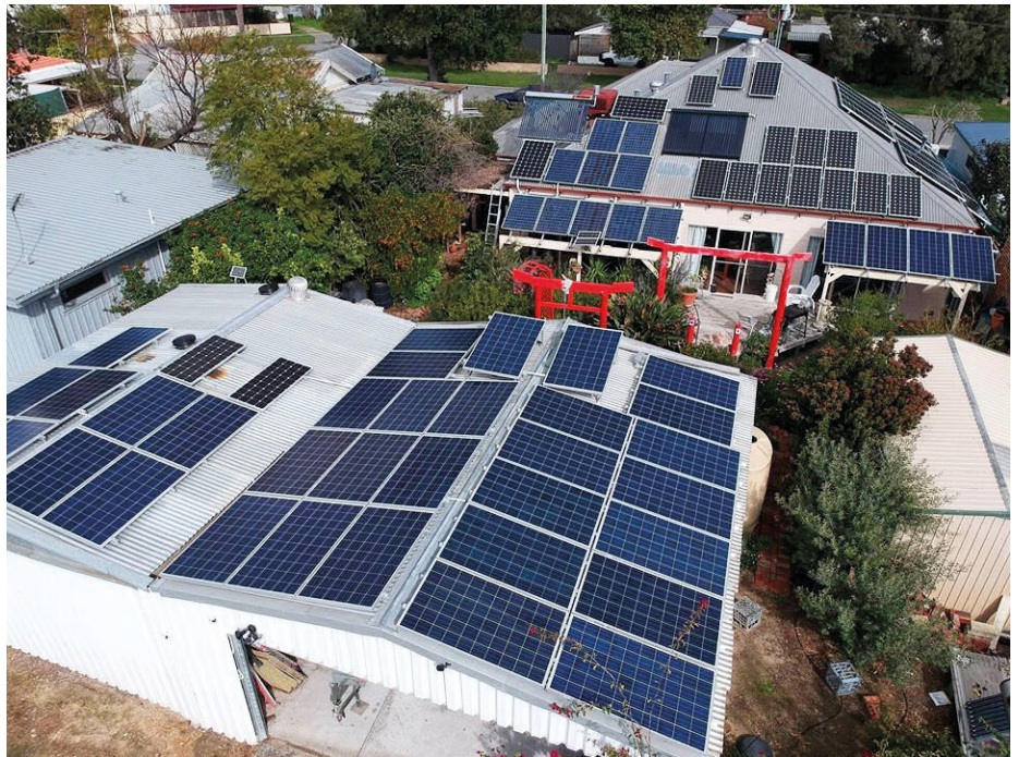
The solar panels on the garage feed power to the house via the Selectronic inverter and the battery bank. As you can see, Martin has quite a few small solar energy systems!
