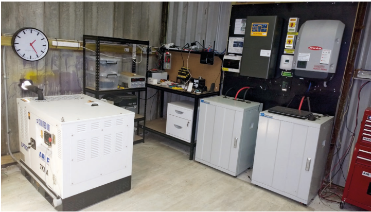
The complete energy system in the back shed. The large box at front left is the diesel generator, the two white boxes at right hold the lithium battery modules. The Selectronic and Fronius inverters can be seen on the wall behind them. The shed uses three-phase power and feeds single-phase power to the house.
